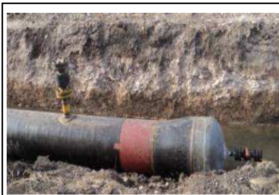
Image 7: IMG Pressure Testing
