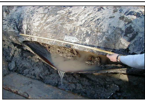
Image 8: IMG Pressure Testing
